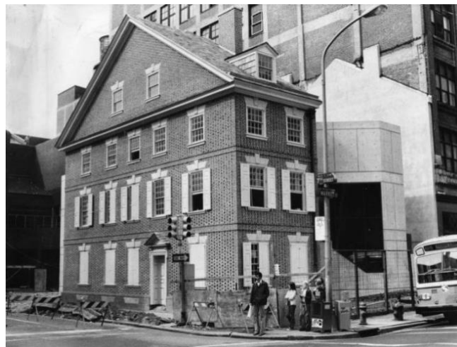
The rebuilt Declaration House upon completion in 1975. | Photo courtesy of Temple University Libraries, Special Collections Research Center
